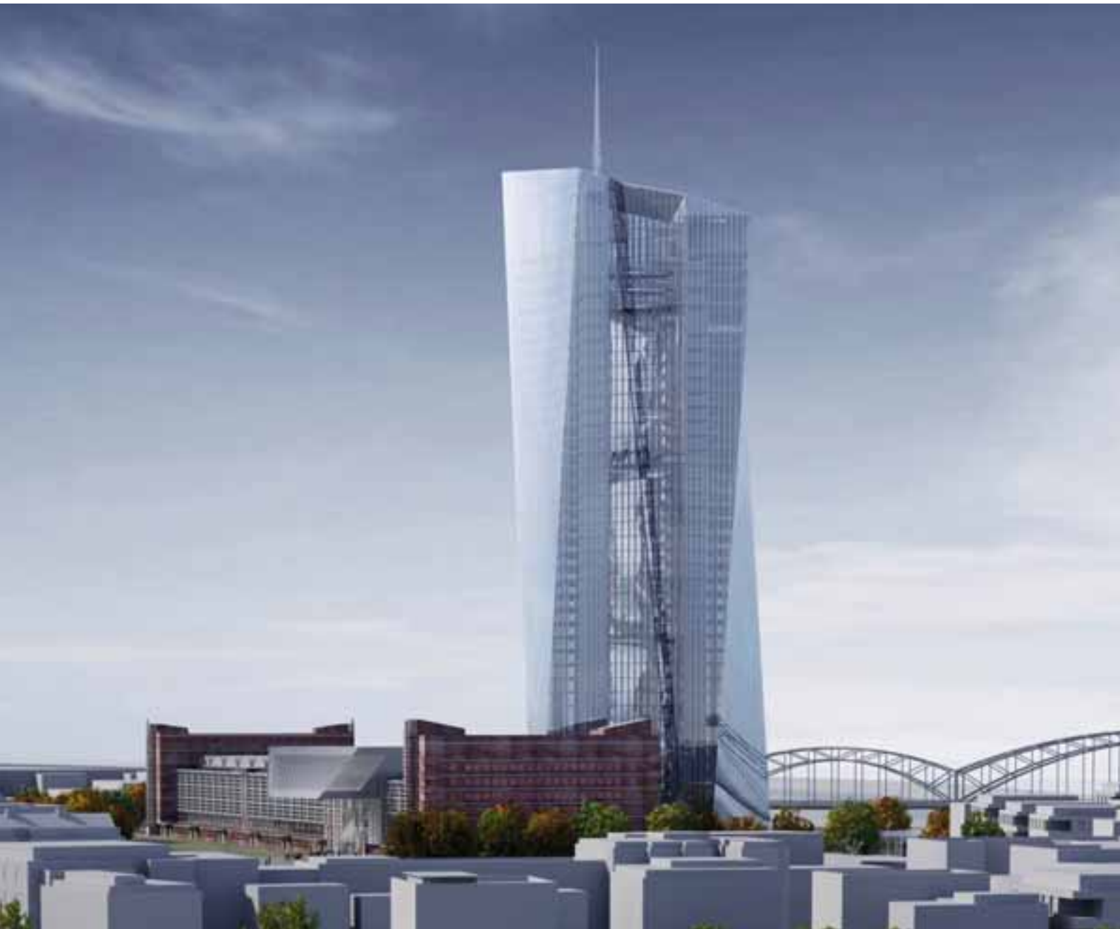
The new ECB premises, designed by COOP HIMMELB(L)AU, are due to be completed by 2013. The ensemble will consist of three main building elements, namely the high-rise, the former Grossmarkthalle and the entrance building.
