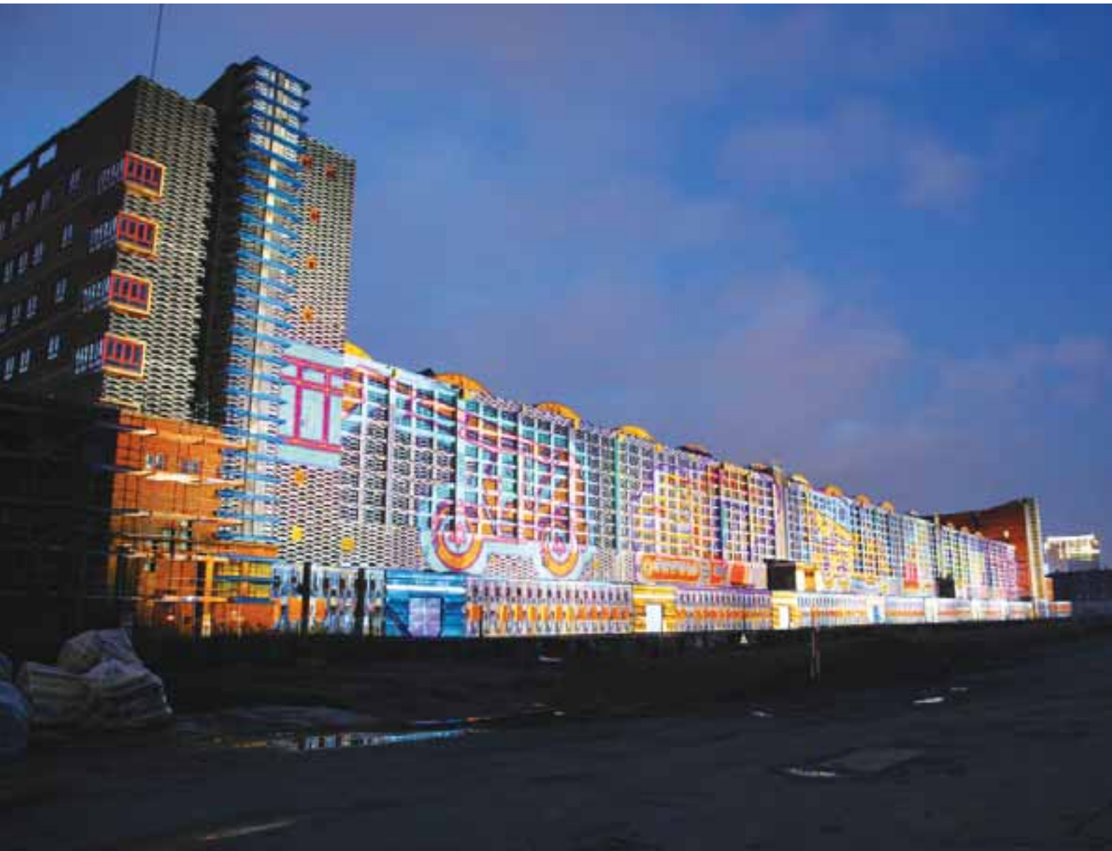
Within the framework of the Luminale 2008, the Grossmarkthalle was illuminated by the lighting artists Casa Magica. This image shows the second of three motifs. It alluded to the upcoming construction works for the new ECB premises.
